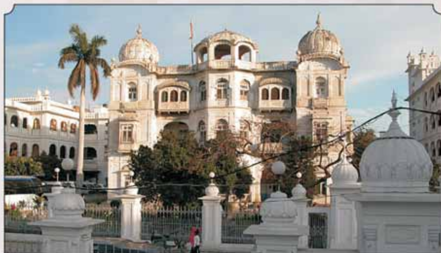
Teja Singh Samundri Hall The Admn. Block of Constitutionally Elected Body of the Sikhs (S.G.P.C.)
